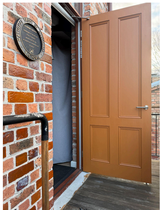
Door to upstairs room (outside view)
