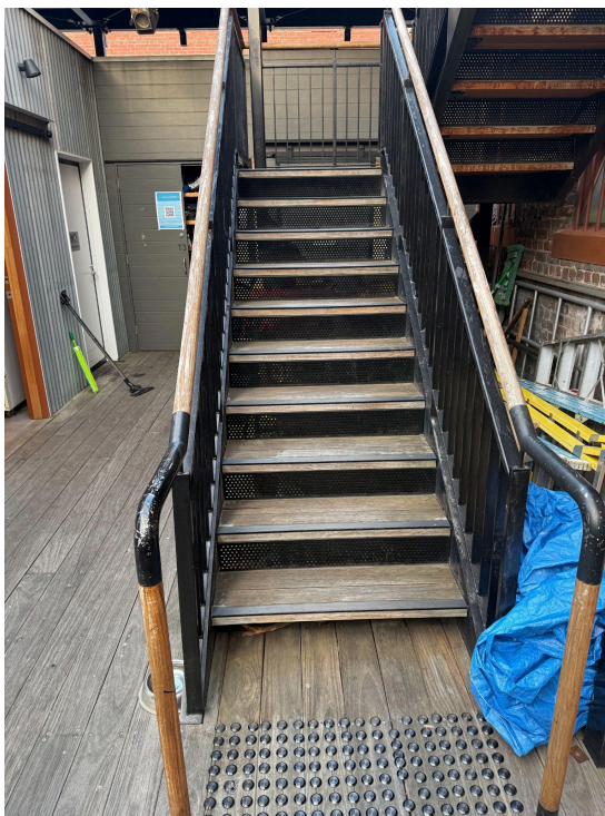
Stairs leading to upstairs room (two flights of stairs)
